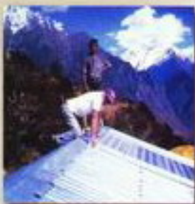
Fitting solar panels at Torge Clinic.
